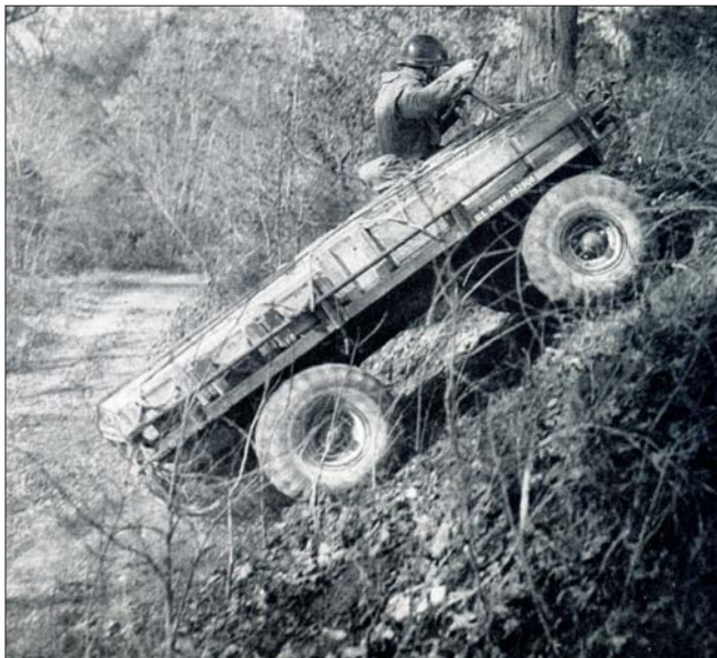
Figure 32. The U.S. Army "Mechanical Mule" magnesium vehicle negotiating rough terrain. 63
